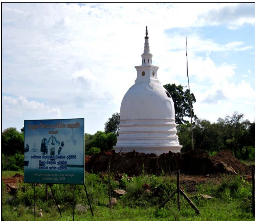
Stupa under construction in Killinochchi.
