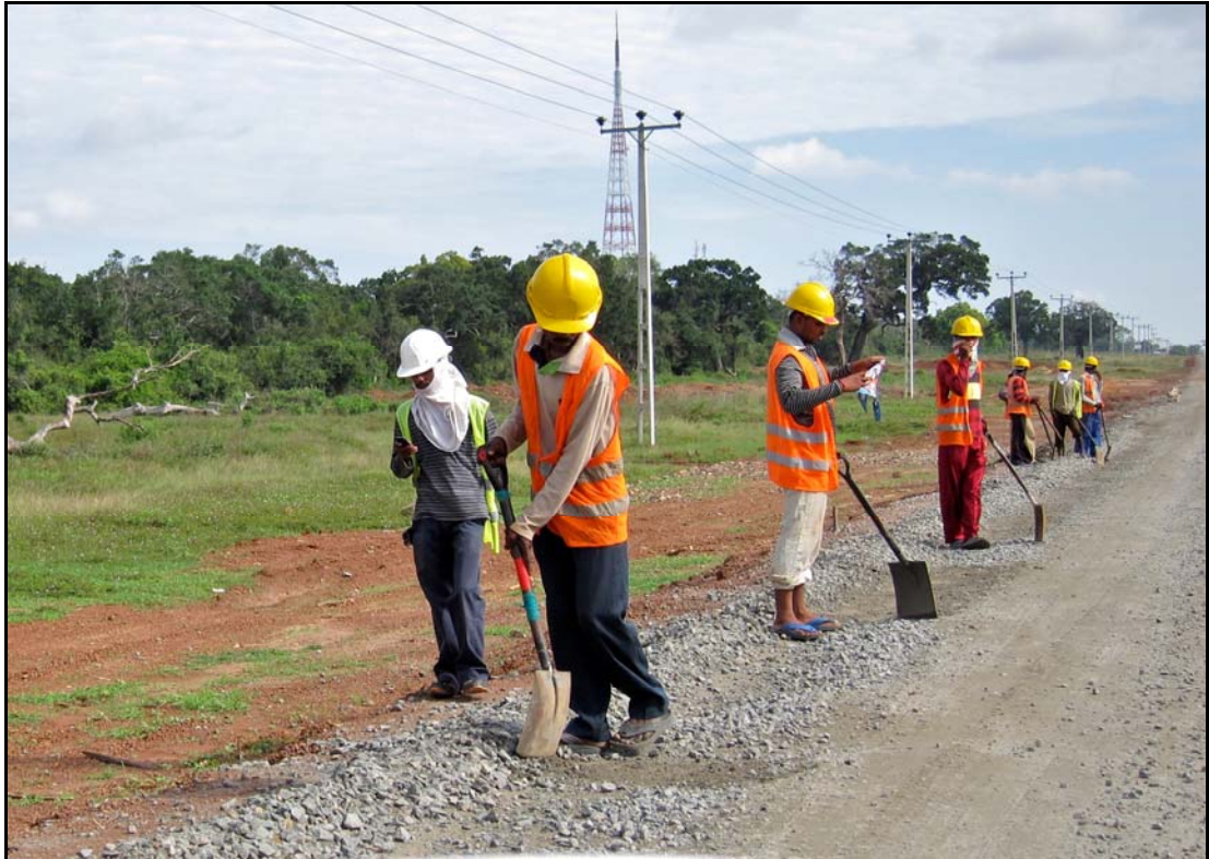
Road workers in Vanni. Tamils from Batticaloa.
