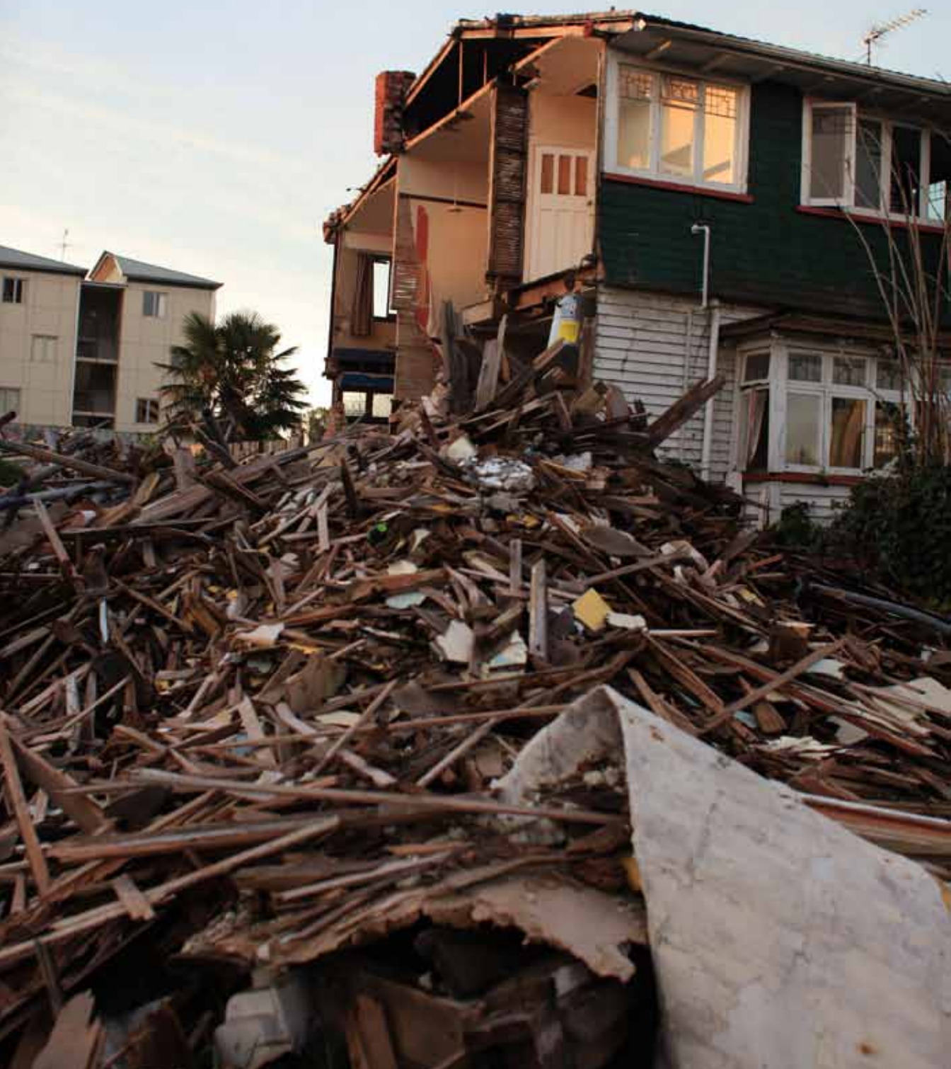
Earthquake damage, Christchurch, New Zealand. Photo: © Alexandra1977 | Dreamstime.com
