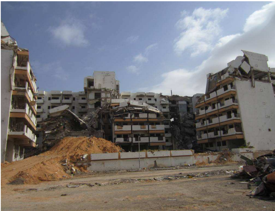
Apartment building struck on 16 September in Sirte © Amnesty International
