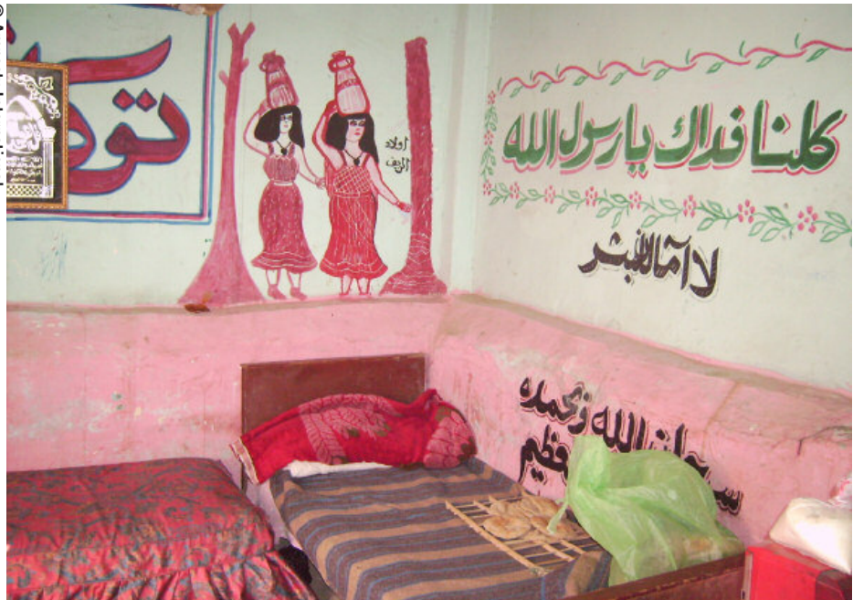
top: The view from the room of Shirihan Hamdi Mohamed Ahmed in Al-Shohba area of Al-Duwayqa, 9 February 2009. She told Amnesty International that the wooden ceiling of her room had collapsed after a rock fall.
