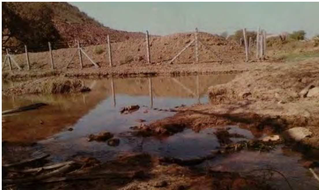
↑ Photo of the spill of liquid taken by a farmer in November 2015. It shows overflow from the perimeter drain.
