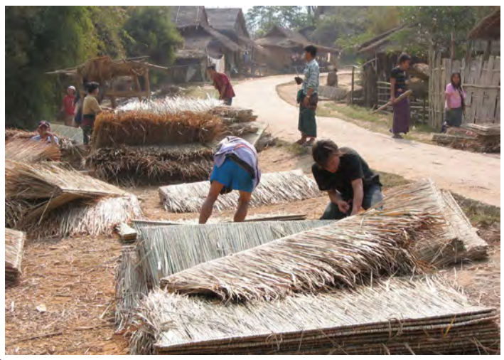
Roofing thatch distribution at Mae La camp
