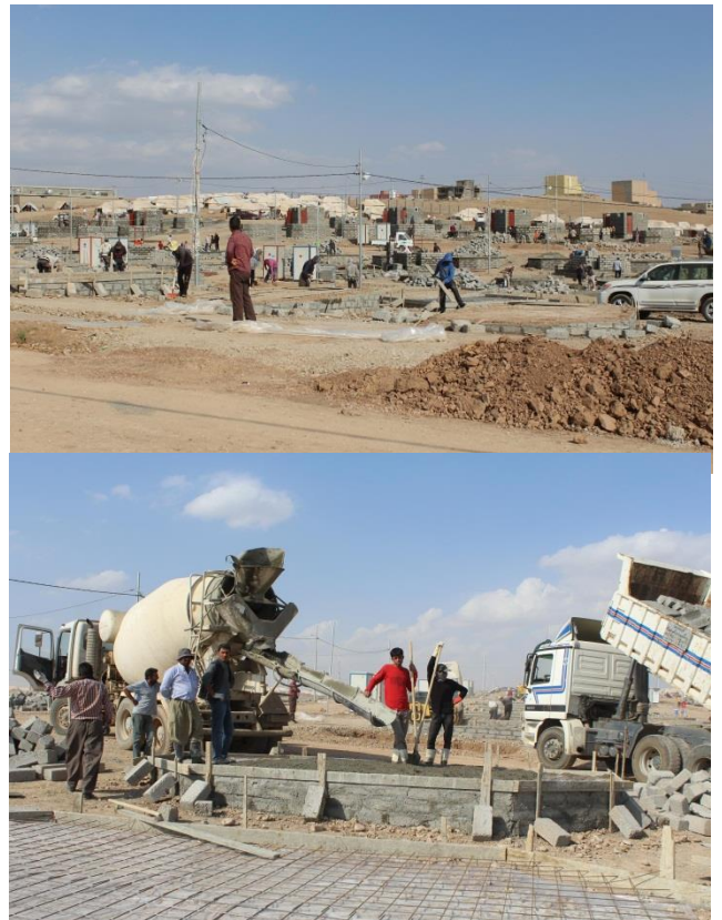
Ongoing construction at Khanke IDP camp, Dohuk governorate. UNHCR/G. Gubaeva.
