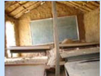
UN-HABITAT - Classroom for rehabilitation
