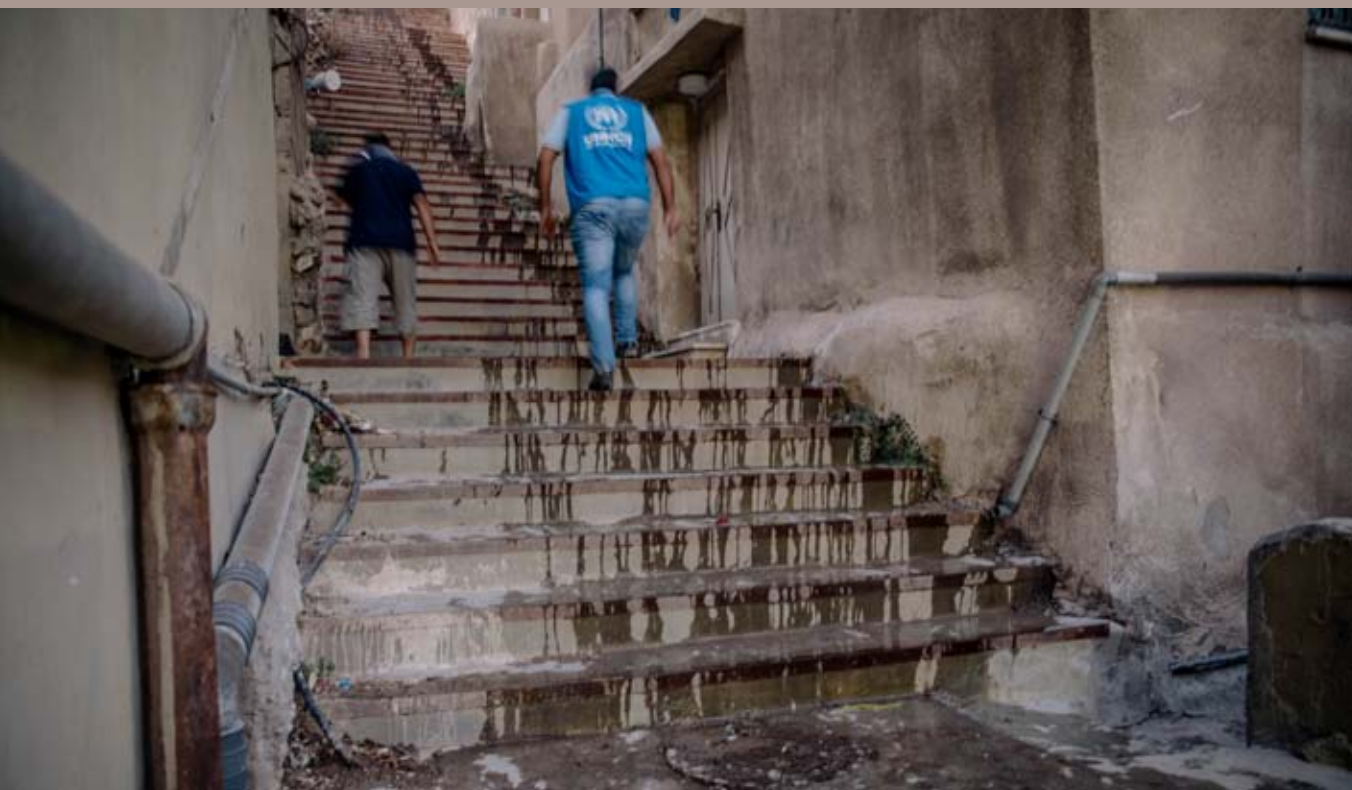
Sewage running down the stairs outside houses occupied by Syrian refugees. ©UNHCR / J. Kohler
