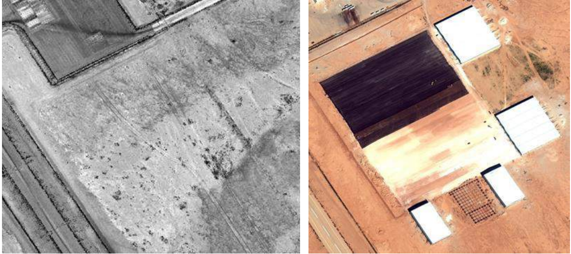
Figure 9 Satellite imagery of Khadim, southern apron area, July 2014 (left) and March 2017 (right): significant engineering work has been carried out to develop a southern apron and increase hangars, suggesting that further air assets are intended to operate from the airbase
