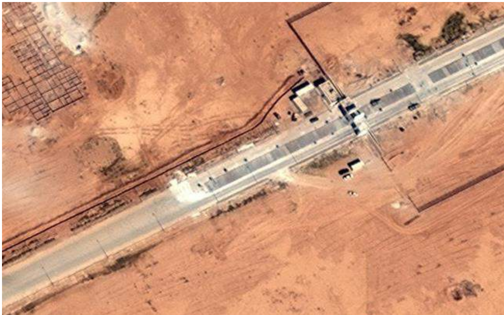
Figure 12 Satellite imagery of Khadim, entrance area, security structure on road, March 2017
