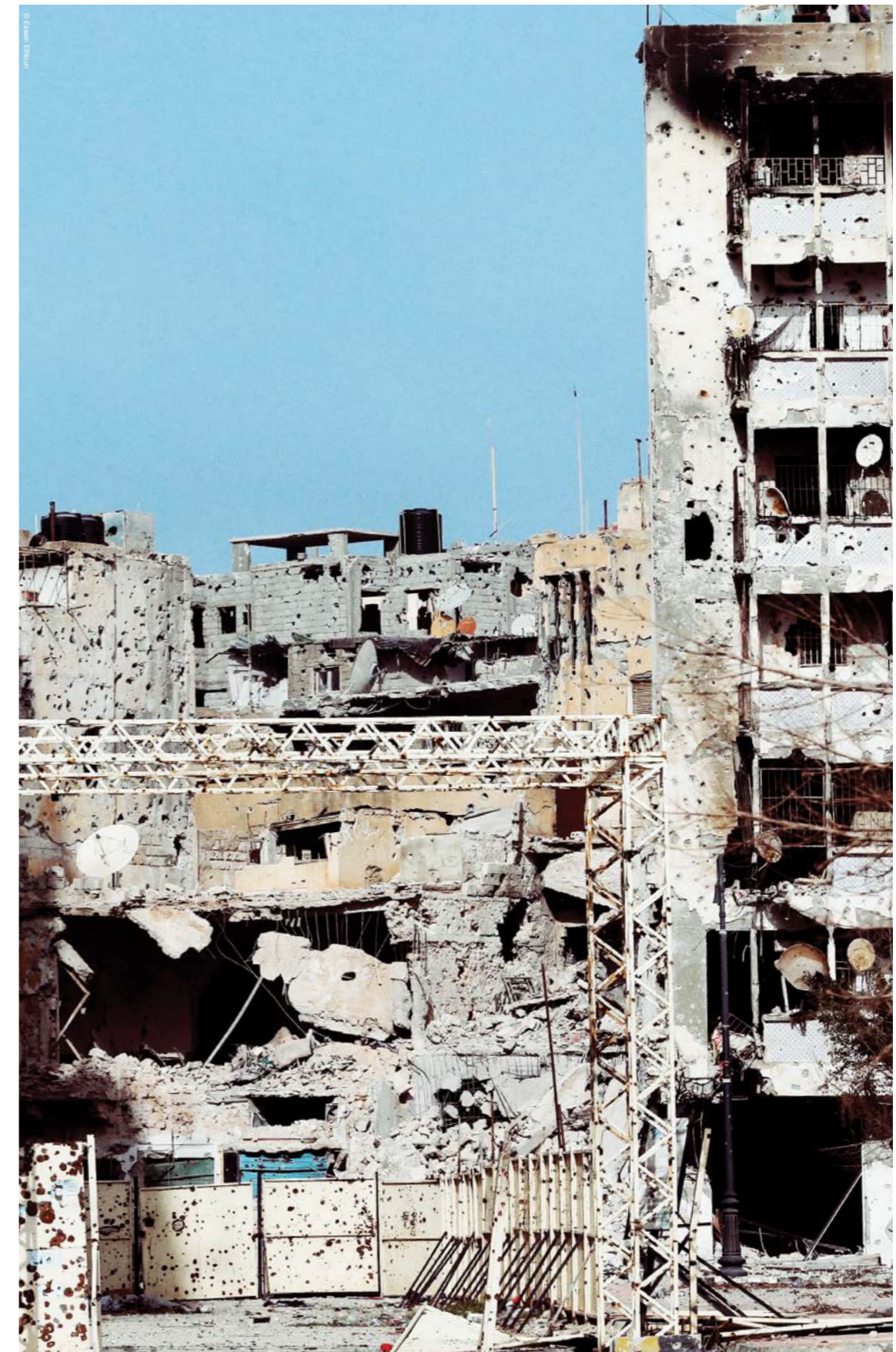
Destruction in the centre of Benghazi as a result of the battle to gain control of the city.
