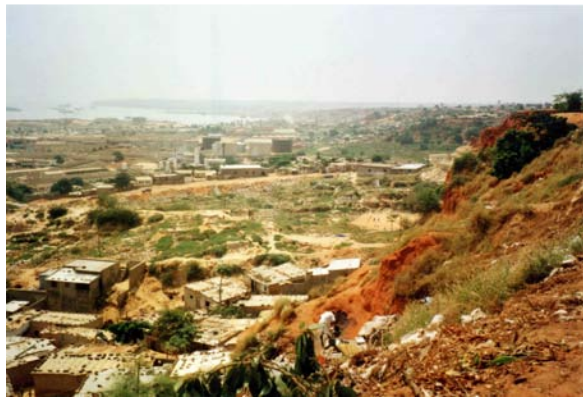
View of Boavista showing the area in which houses were demolished. © AI, May 2003
