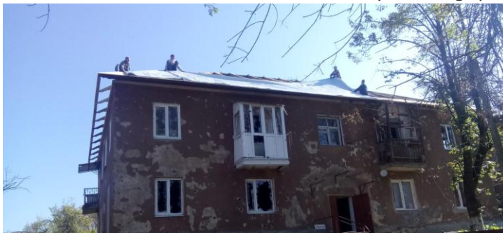
88 households in Semenivka in neighborhood of Slovyansk received reinforced tarpaulin from UNHCR for fast roofing repairs
