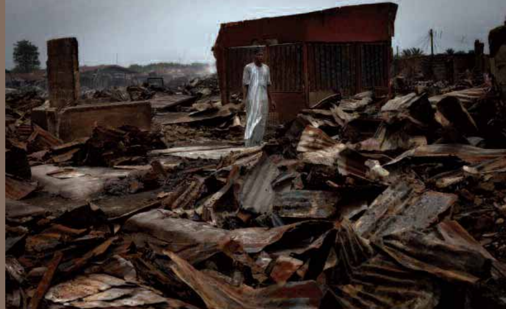
(above) A man stands in the rubble of the main market in Kafanchan, Kaduna State, on April 25, 2011. Hundreds of shops, houses, and vehicles were burned during the April 18-19, 2011 violence in Kafanchan.
