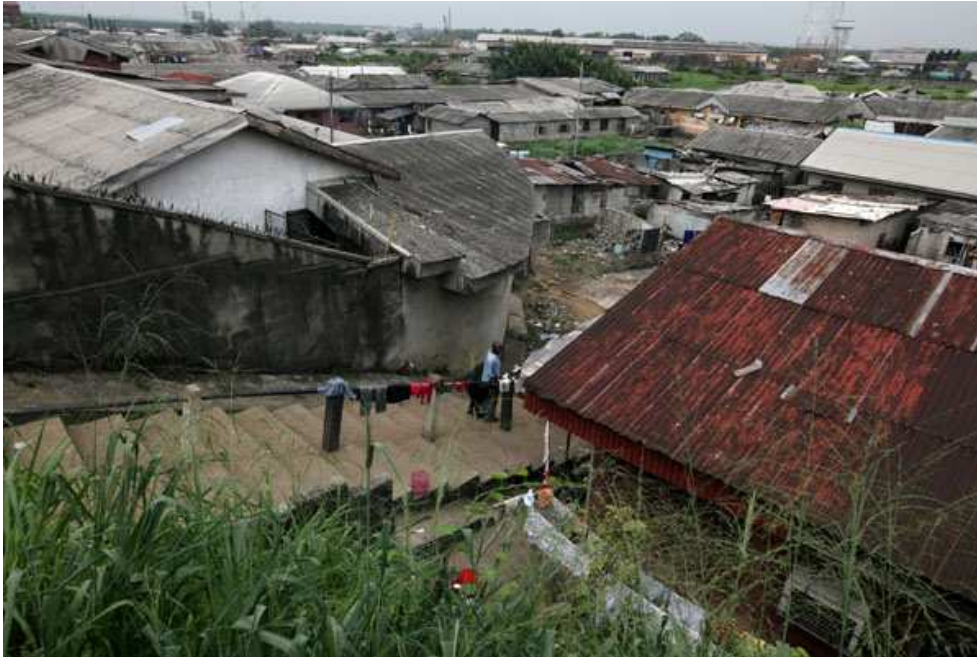
Abonnema Wharf before the demolition – 27 April 2011
