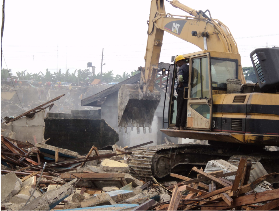
Bulldozer demolishing houses in Abonnema Wharf – Thursday 28 June 2012
