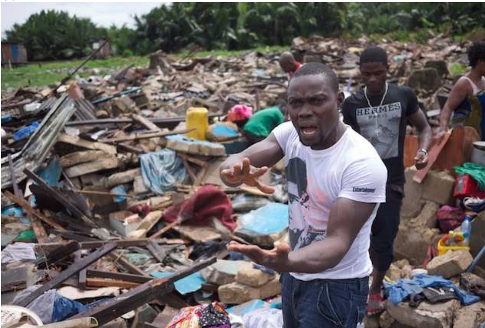
A former resident in Abonnema Wharf expressing anger at the demolitions on day 1, Wednesday 27 June 2012
