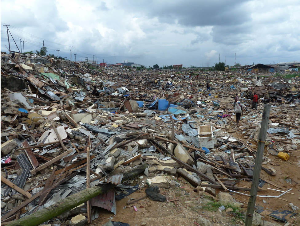
Abonnema Wharf, now a sea of rubbles after five days of demolitions in the community - Sunday 1 July 2012
