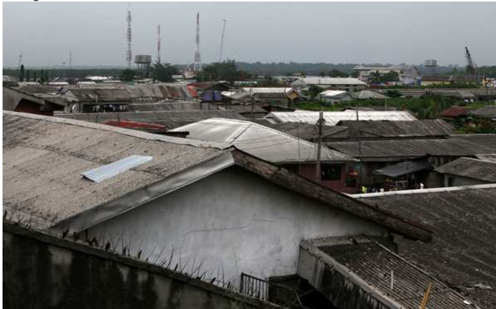
What Abonnema Wharf looked like before the demolitions -27 April 2011
