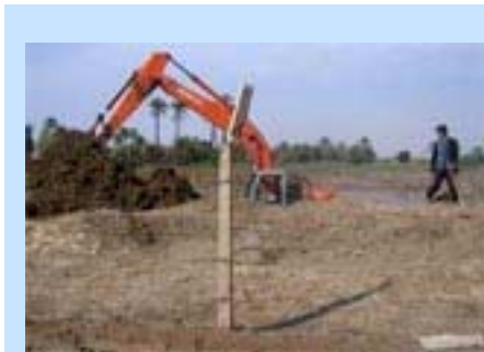
Clearing access routes - UNHCR
