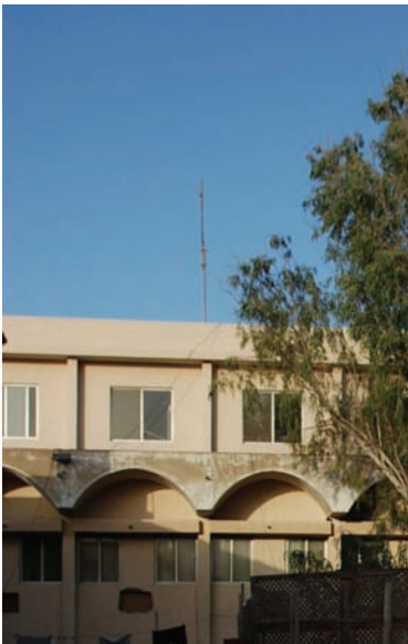
Rear view of the Karachi headquarters of the Intelligence Bureau. An individual, referred to as "ZZ" in this report, was allegedly detained and tortured in this building. It is walking distance from the British Deputy High Commission in Karachi. © 2009 Private
