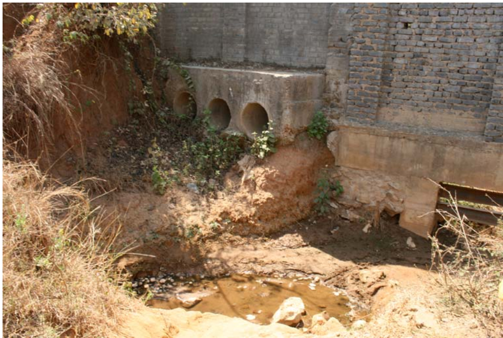
Photo 14: Drainpipe at the refinery's boundary wall near the river at Chhattarpur (Amnesty International)
