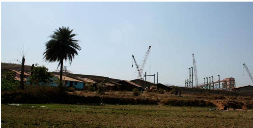
Photo 17: The Lanjigarh refinery's boundary wall, barely 150 metres away from Bandaguda village (Amnesty International)
