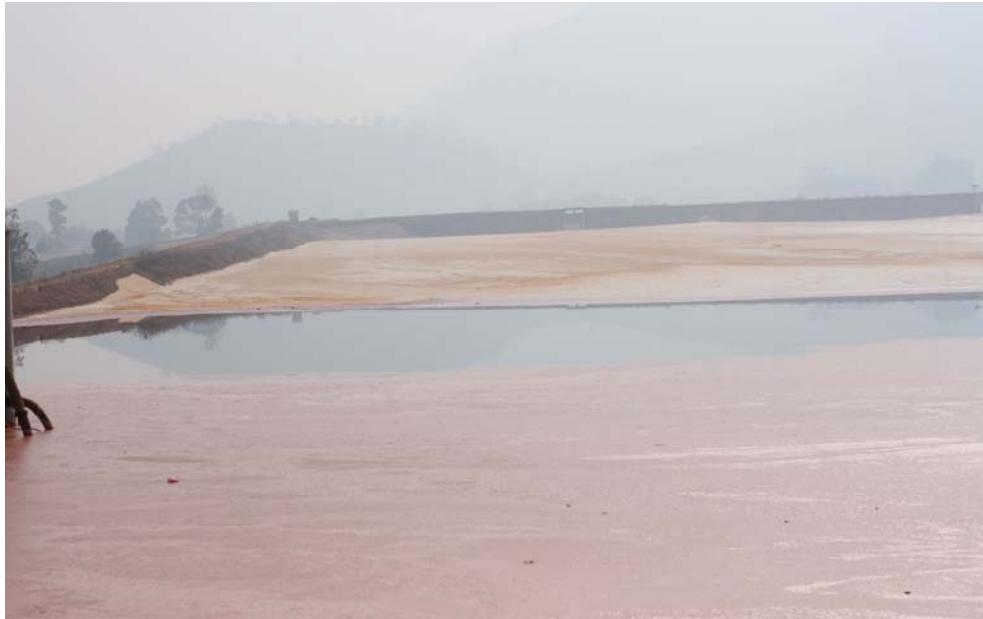
Photo 11: A view of the refinery's red mud pond at Lanjigarh (Amnesty International)
