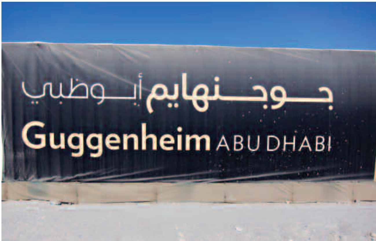
The construction site of Guggenheim's Abu Dhabi branch, which is now expected to open in 2017.
