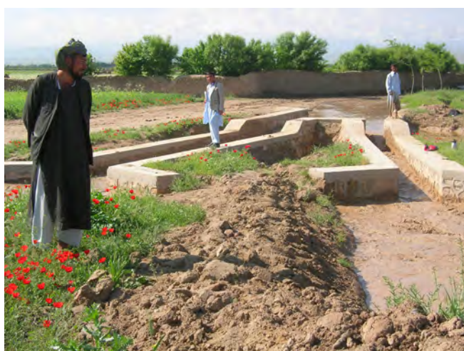
Image 7: Proportional divider, Wulayat canal, Sar-i-Pul Province
