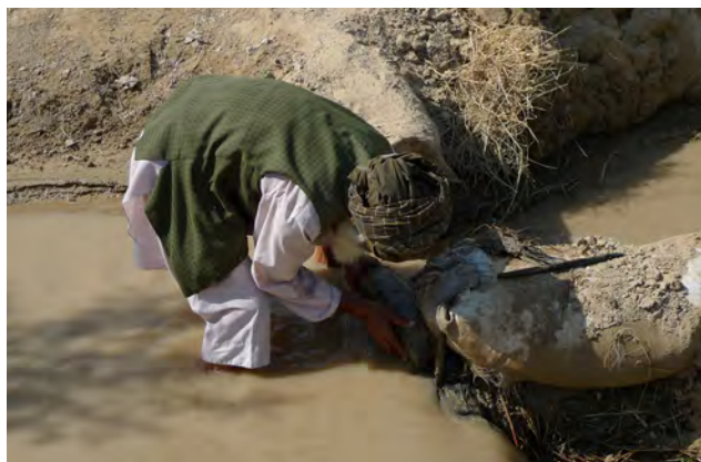
Image 15: A canal mirab re-adjusting a jui divider that has been tampered with.
