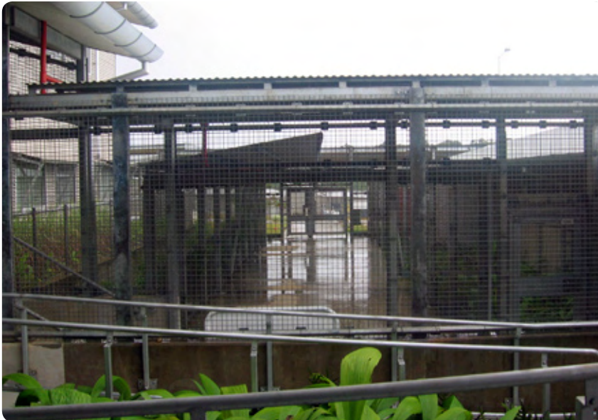
..... Caged walkways, Christmas Island IDC
