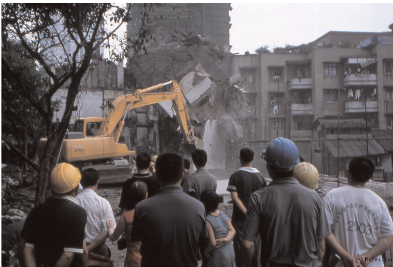
A building demolition in the district of Jiaochangkou, 2005.
