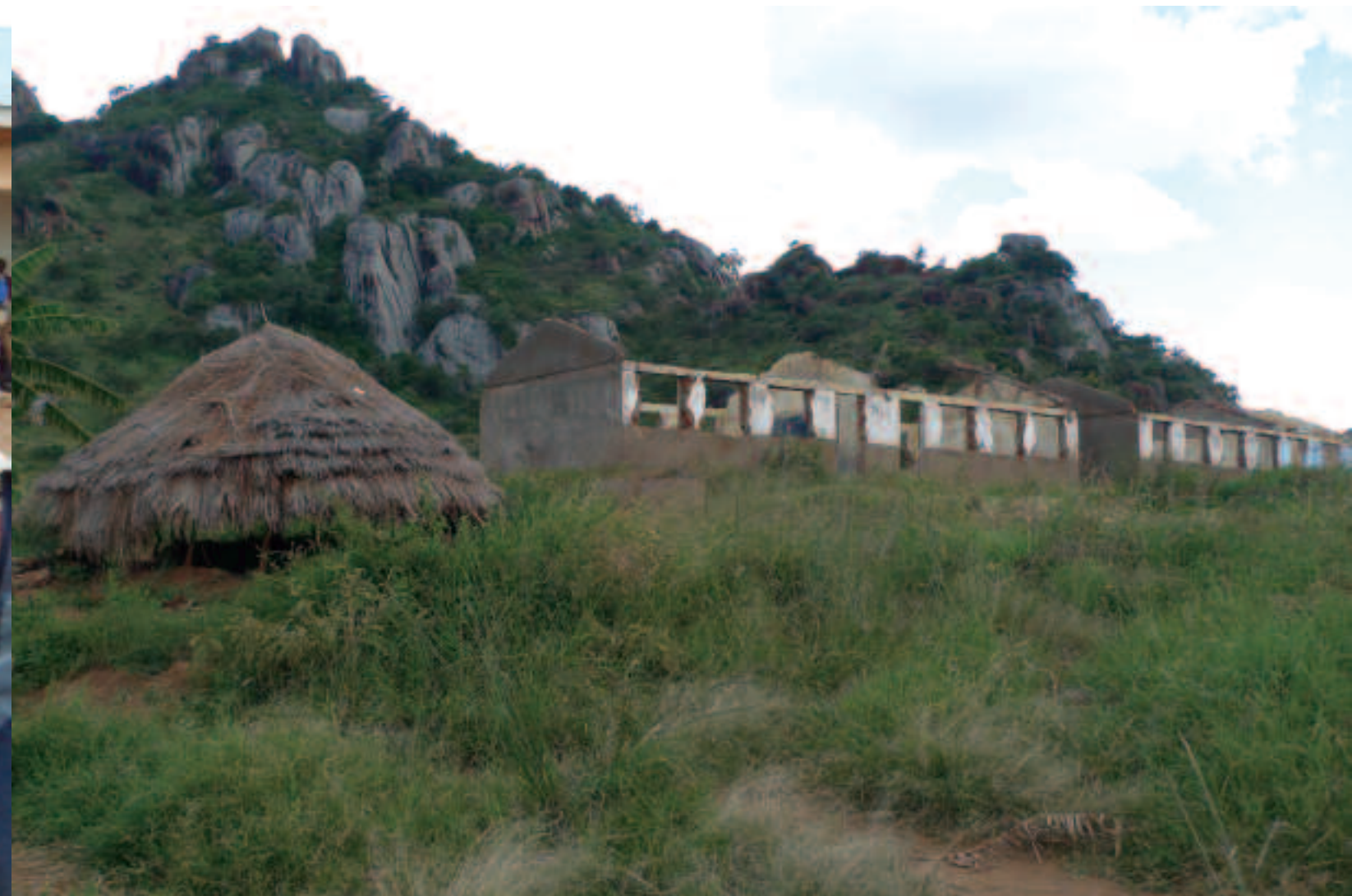
A dilapidated school, Lopedo, Kaabong.
