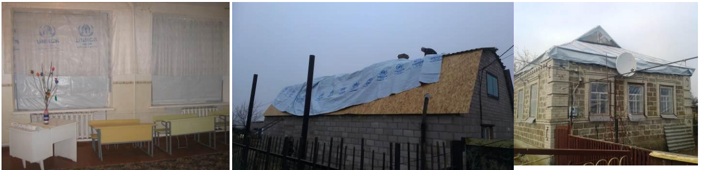
UNHCR continues to distribute reinforced plastic sheets to affected villages and towns. During the last week, despite ongoing hostilities, people in Talakovka in southern Donetsk region managed to cover the damaged parts of their homes, schools and kindergartens.
