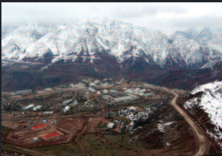
A construction site for the proposed Rogun Dam.
