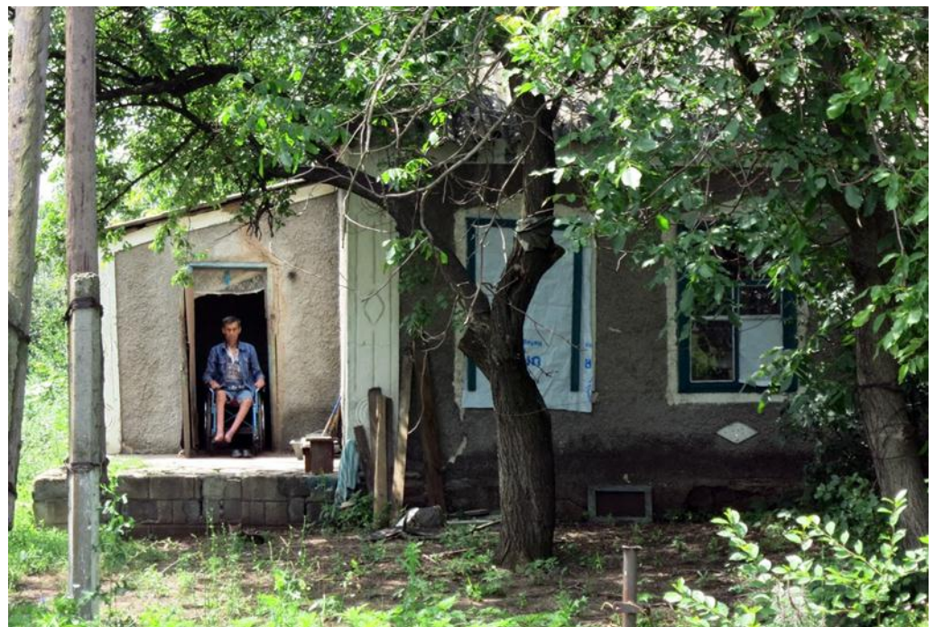
A disabled man sits at the porch of his damaged house in Granitnoye, a small village next to Mariupol. Due to ongoing clashes, the frontline village has many buildings destroyed and suffers from infrastructure and water supply disruptions. Although many residents fled Granitnoe, some people decided to stay. UNHCR provided reinforced tarpaulin to cover broken windows and roofs to the most vulnerable residents of Granitnoe. Photo: UNHCR/I.Bulgakov
