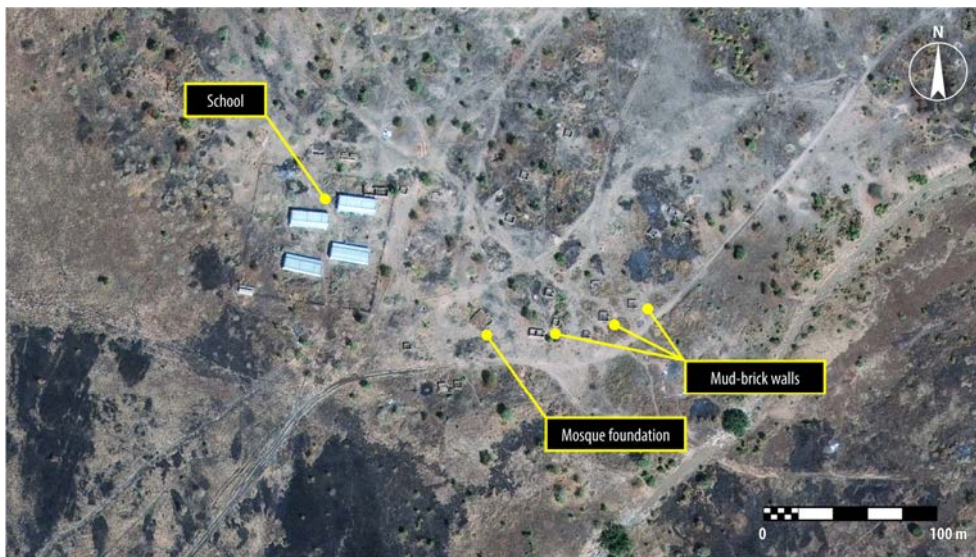
Figure 18: Only the school buildings remained standing in Jegu on 25 January 2013
