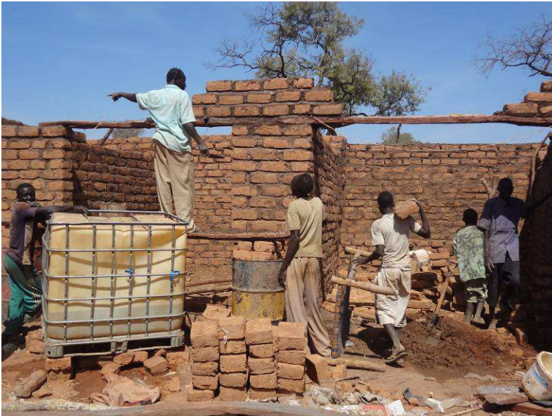
Construction in Yida's market by the refugee population, January 2013 © Amnesty International
