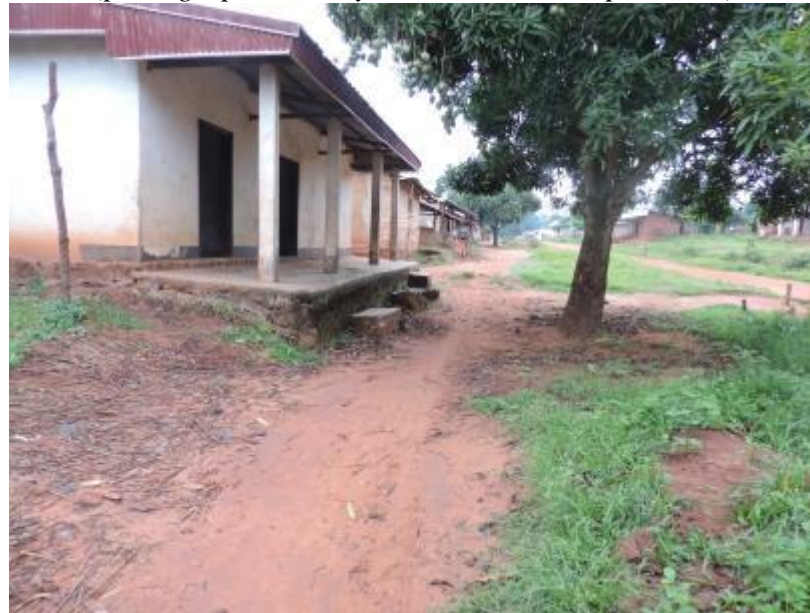
House that came under siege by anti-Balakas during the attack on Guen (photograph taken by the Panel on 26 April 2014)
