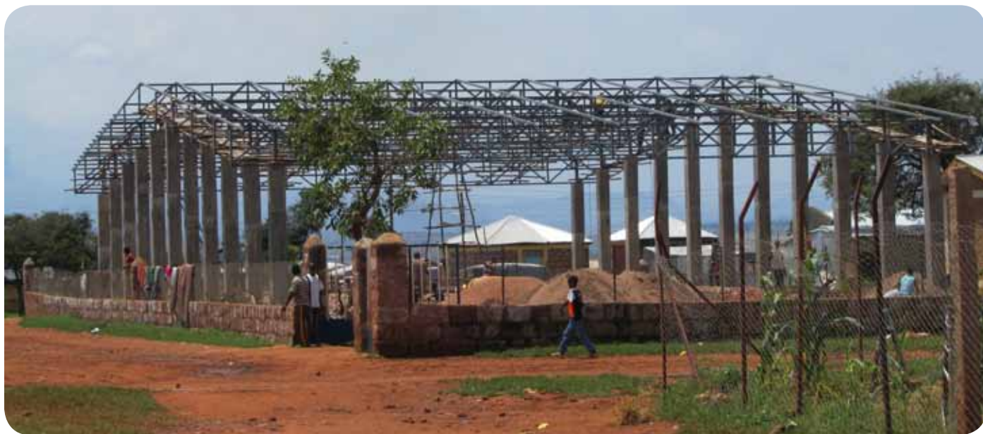
JRS sports and social center under construction in Mai-Aini Camp.
