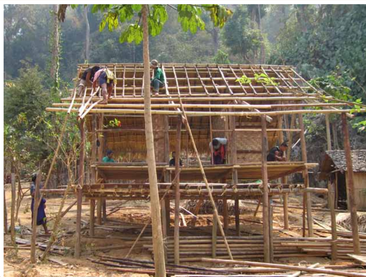
House construction at Site 1
