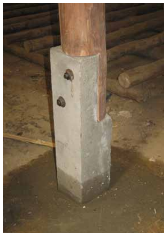
Concrete post foundations
