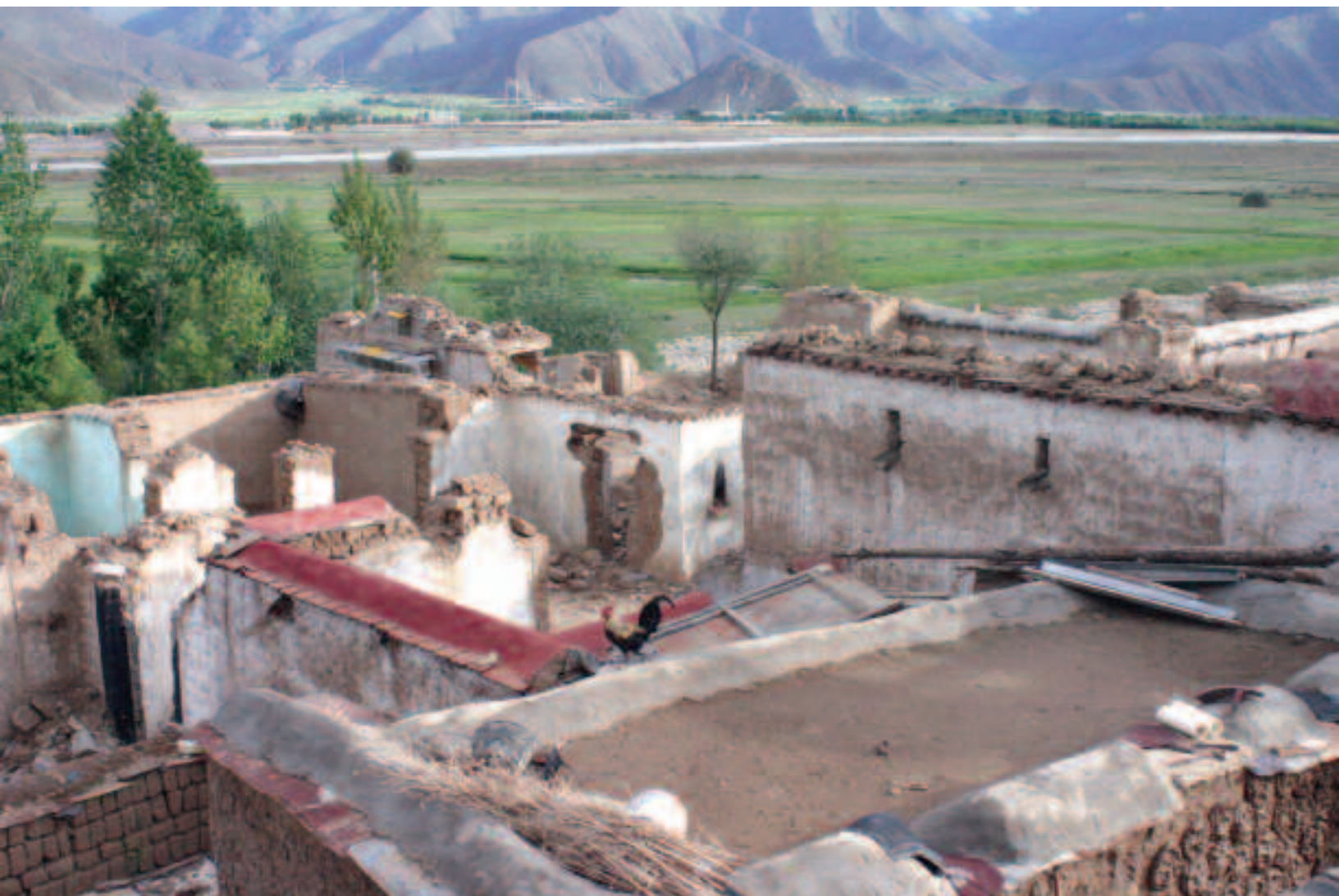
Old houses being dismantled at Garpa, Tibet Autonomous Region.
