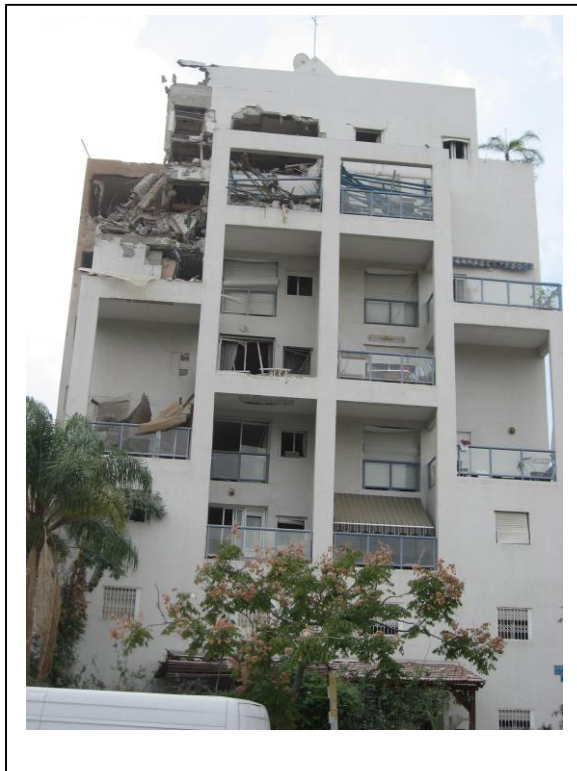
Damage to apartment buildings in Rishon LeZion caused by a rocket fired on 20 November 2012 from the Gaza Strip, during the eight-day Israel/Gaza conflict. © Amnesty International
