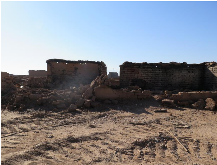
Fresh Bulldozer tracts visible next to destroyed homes in Umm Khabari
