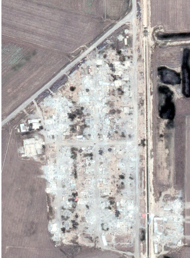
Nahrawan is completely destroyed © CNES, Distribution AIRBUS DC
