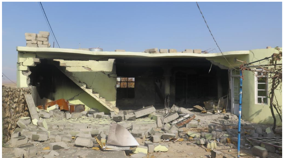
Destroyed house in Barzanke © Amnesty International
