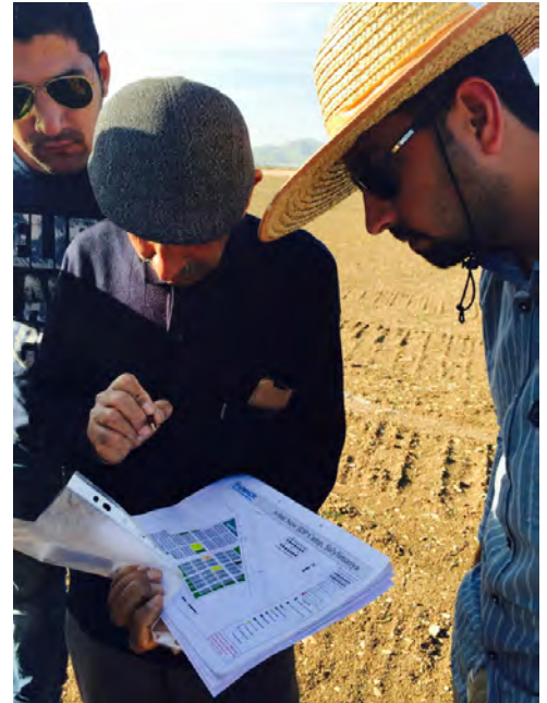
UNHCR site planner oversees the construction of Ashti Camp, Sulaymaniyah Governorate, designed to accommodate some 6,000 people (UNHCR/ D. Tilakamonkul)
