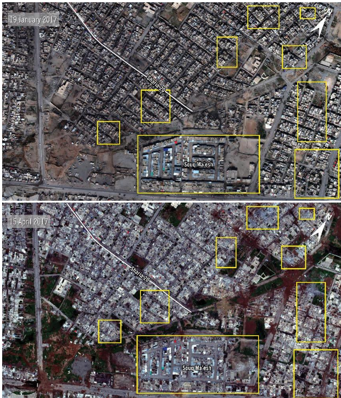
Major damage is visible in the al-Tenak neighbourhood near Souq Ma'esh between 19 January 2017 and 15 April 2017. Areas with significant damage are highlighted with yellow boxes. Image: © 2017 DigitalGlobe, Inc.
