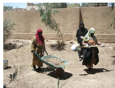
Rehabilitating a public building. Photo: WFP
