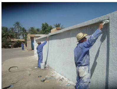
Rehabilitating a public building. Photo: WFP
