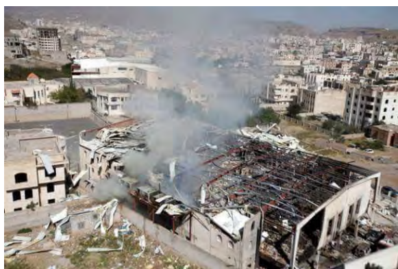
Figure 49.D.2 Post blast aerial image 298
