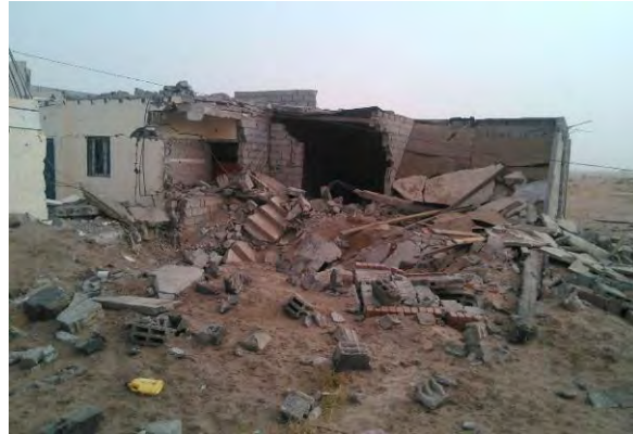
Figure 49.B.3 Armed group suspect's house post-explosion
