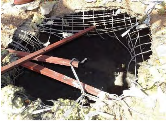
Figure 49.D.4 Entry point EO1
