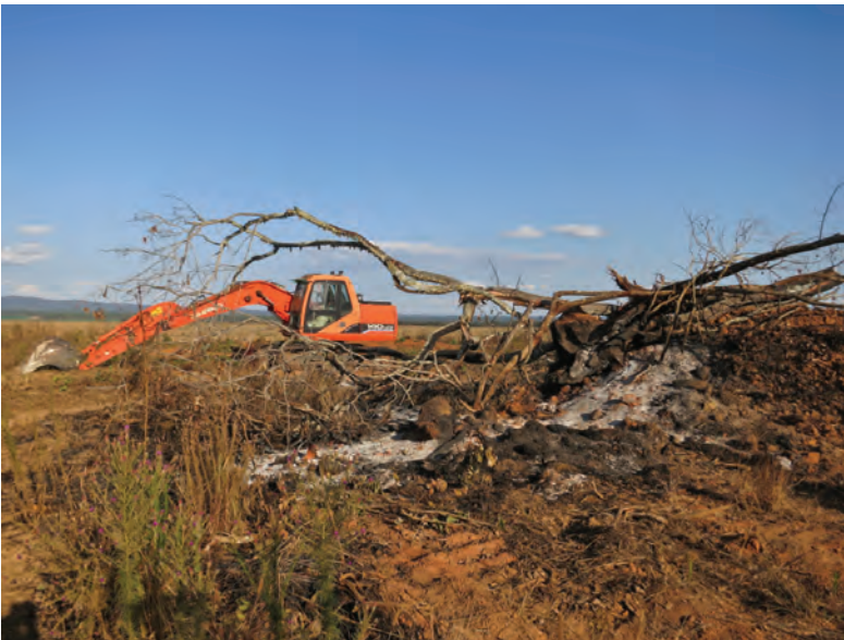
(above) Excavator used to clear land on a commercial farm in Luombwa farm block, Serenje district, after long-term rural residents were displaced.
