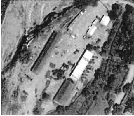
Tank base in Buzala, 2008
