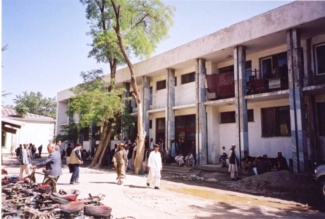
Kabul Welayat - one of the two main courts in Kabul. It houses some of the primary city courts, family court and public security court. ©AI
