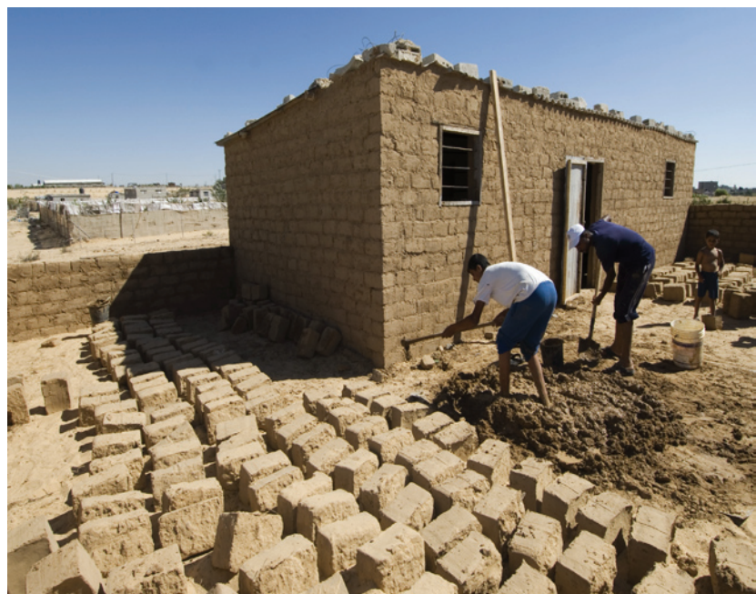
House constructed with mud bricks, Rafah. June 2009.
