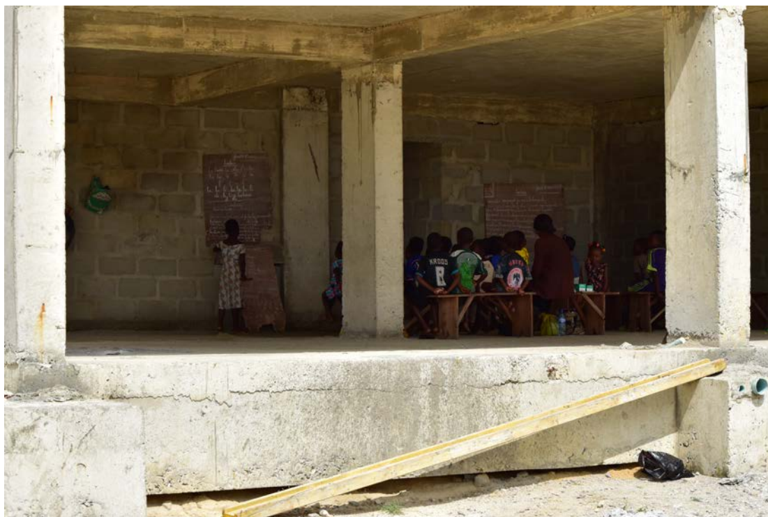
Ilubirin children taking lessons in one of the government's under-construction buildings. The classes moved here after the school it was demolished in November 2015. 19 May 2016
