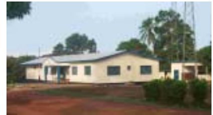
Rehabilitated Kambia Police Station
