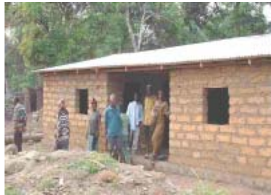
Newly constructed building in Kono District
