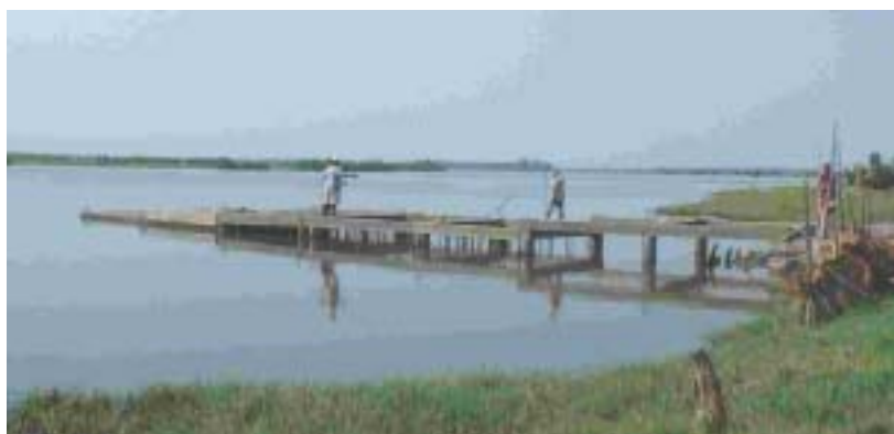
Jetty under construction: Rosinor, Kambia District
