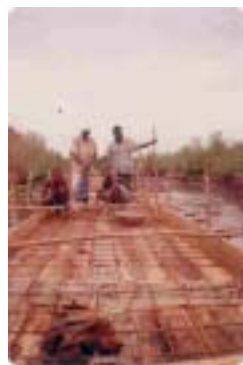
Bridge building in Bonthé
