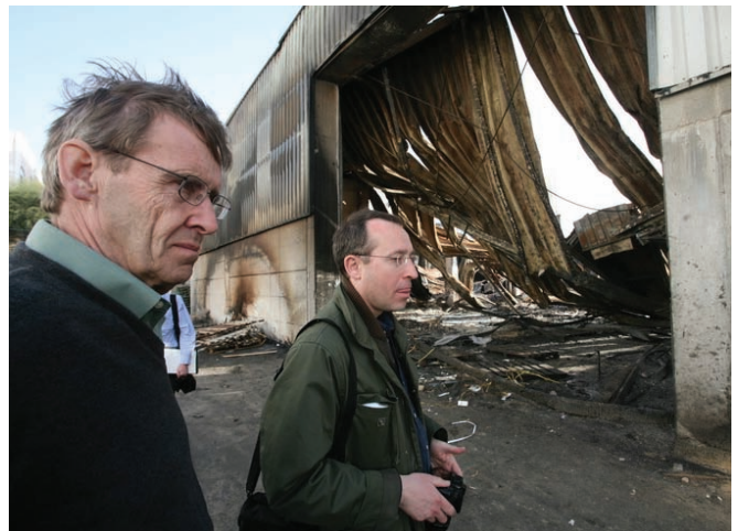
Martin Linton MP and Andy Slaughter MP at the damaged UN warehouse, UNRWA headquarters, Gaza City
