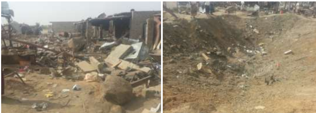
Figure II Damage to the Khamees market
