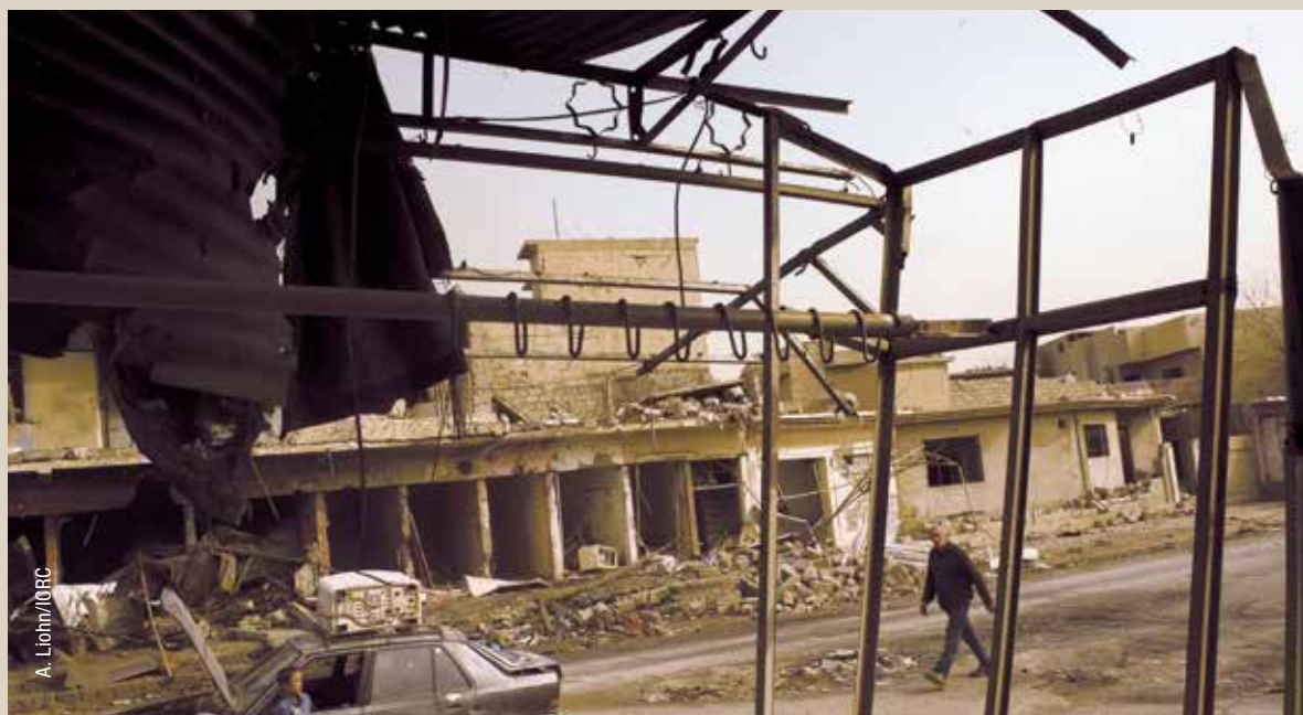
Damaged residential area in eastern Mosul. February 2017.
