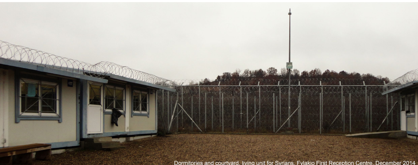
Dormitories and courtyard, living unit for Syrians, Fylakio First Reception Centre, December 2014
