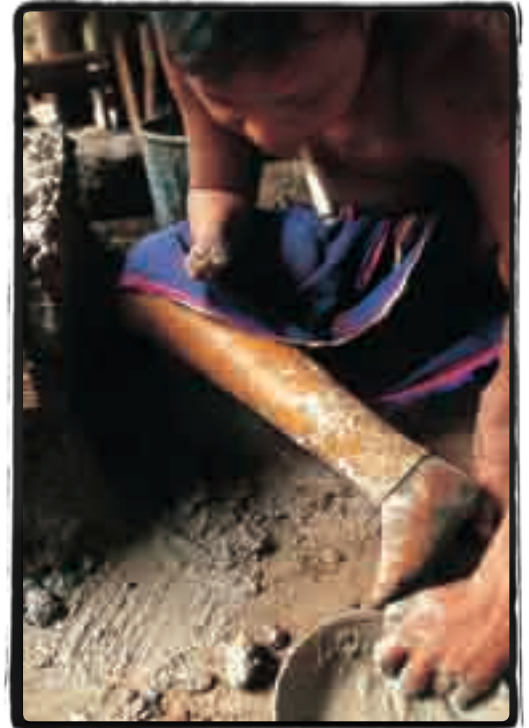
(Above) Working on construction in Mae Ra Ma Luang camp.
