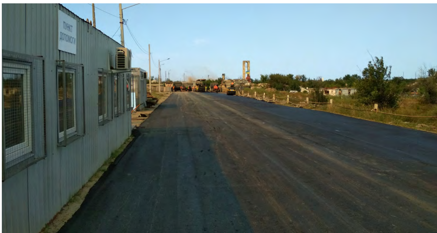
Stanytsia Luhanska EECP, Asphalt road reconstruction
